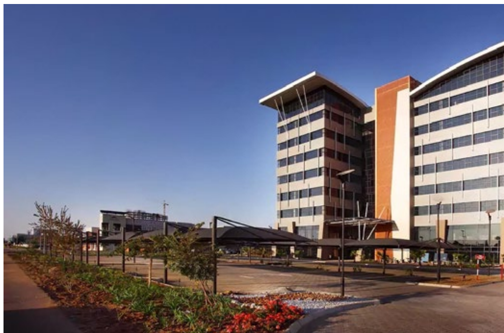
From diamond wealth to national development. The discovery of diamonds transformed Botswana's fiscal future, financing an ambitious programme of infrastructure development that connected the nation through modern roads, expanded electricity generation and transmission, built schools and hospitals, and laid the physical foundations for one of Africa's most remarkable development stories.
